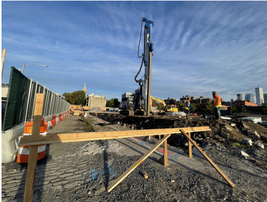
Photo 1: Kingdom installing a soldier pile in the southern part of Society Brooklyn (facing northwest)
