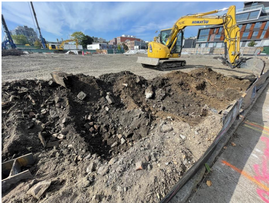
Photo 2: Kingdom excavating in the northern part of Society Brooklyn to pre-clear obstructions prior to SOE installation (facing southwest)
