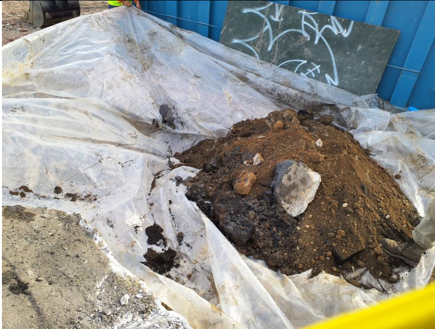
Photo 3: Soil/fill impacted during floor drain removal, stockpiled on top of polyethylene sheeting in the northwestern part of Society Brooklyn (facing northeast)
