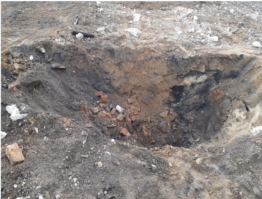
Photo 4: View of the completed floor drain over-excavation in the northwestern part of Society Brooklyn (facing northeast)
