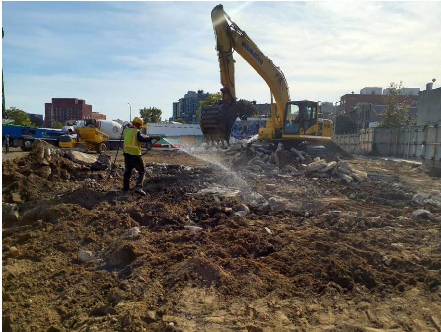
Photo 1: Kingdom using water to suppress dust while excavating in the northwestern part of Society Brooklyn (facing south)
