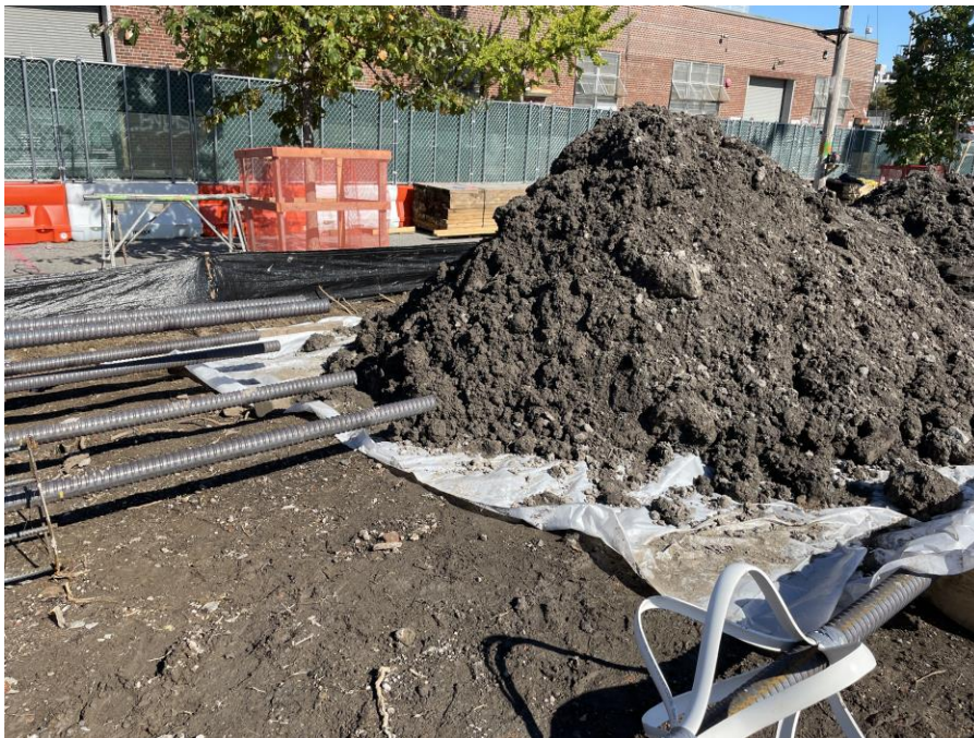
Photo 2: Kingdom stockpiling drilling spoils in preparation for future off-site disposal in the northeastern part of Society Brooklyn (facing northeast)
