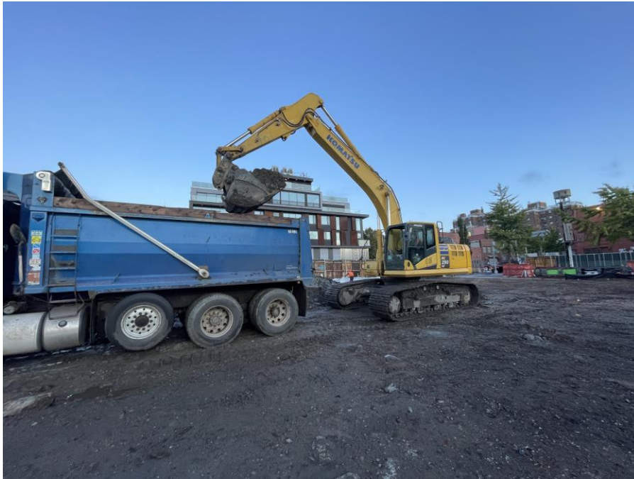
Photo 1: Kingdom loading a permitted tri-axle truck with non-hazardous soil for off-site disposal from Society Brooklyn (facing west)
