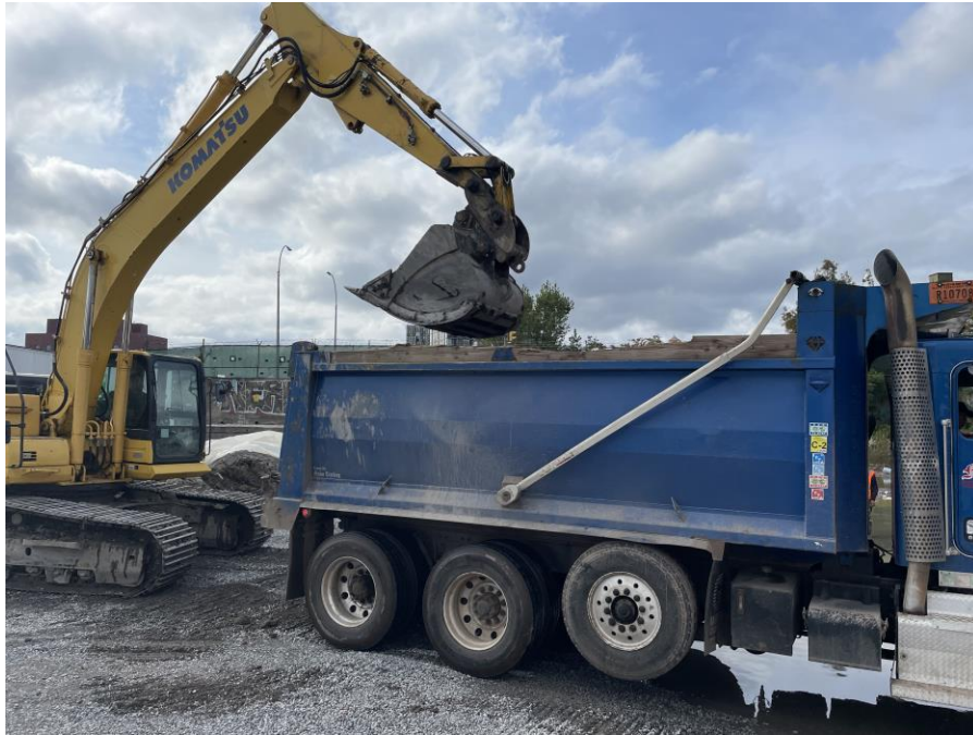
Photo 1: Kingdom loading a permitted tri-axle truck with non-hazardous drilling spoils for off-site disposal from Sackett Place (facing southwest)
