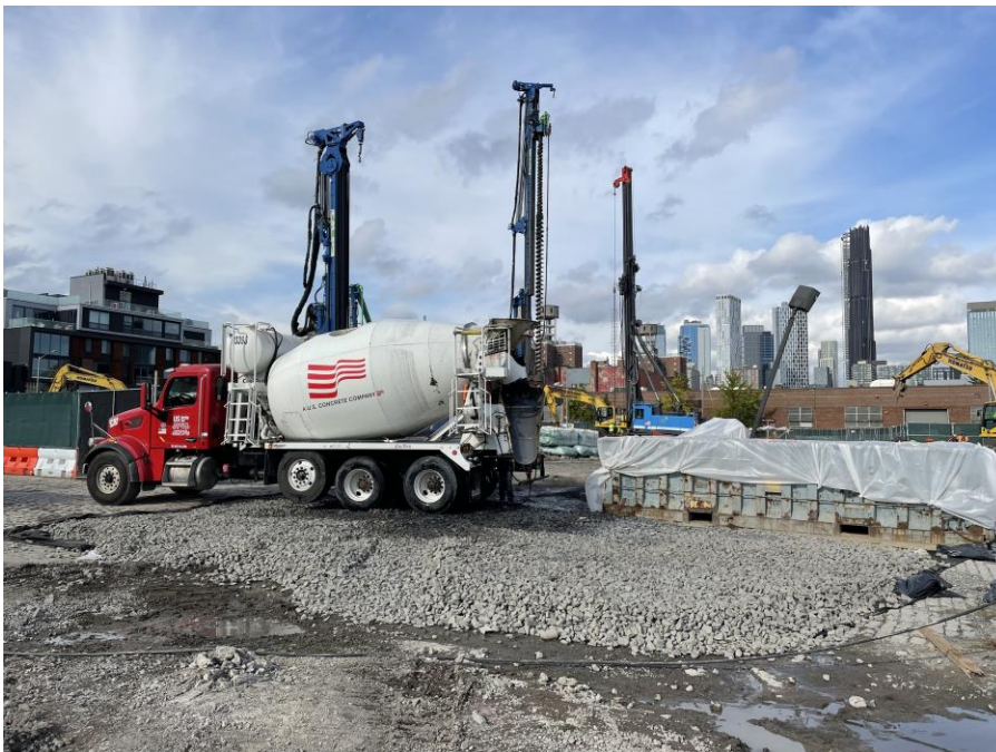
Photo 2: Concrete truck using the newly constructed stabilized construction entrance (facing northwest)
