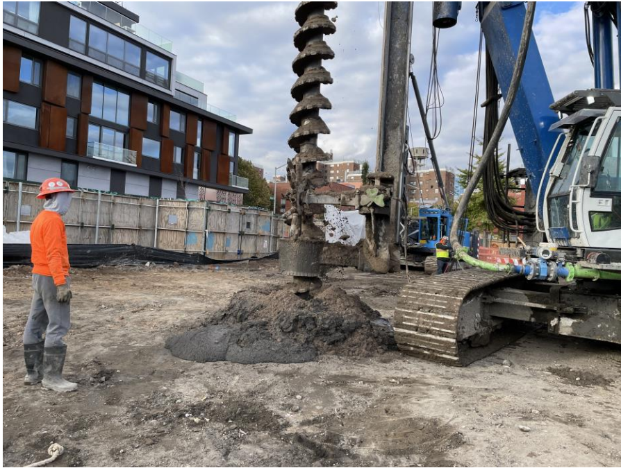
Photo 1: Kingdom installing a foundation pile in the western part of Society Brooklyn (facing northwest)
