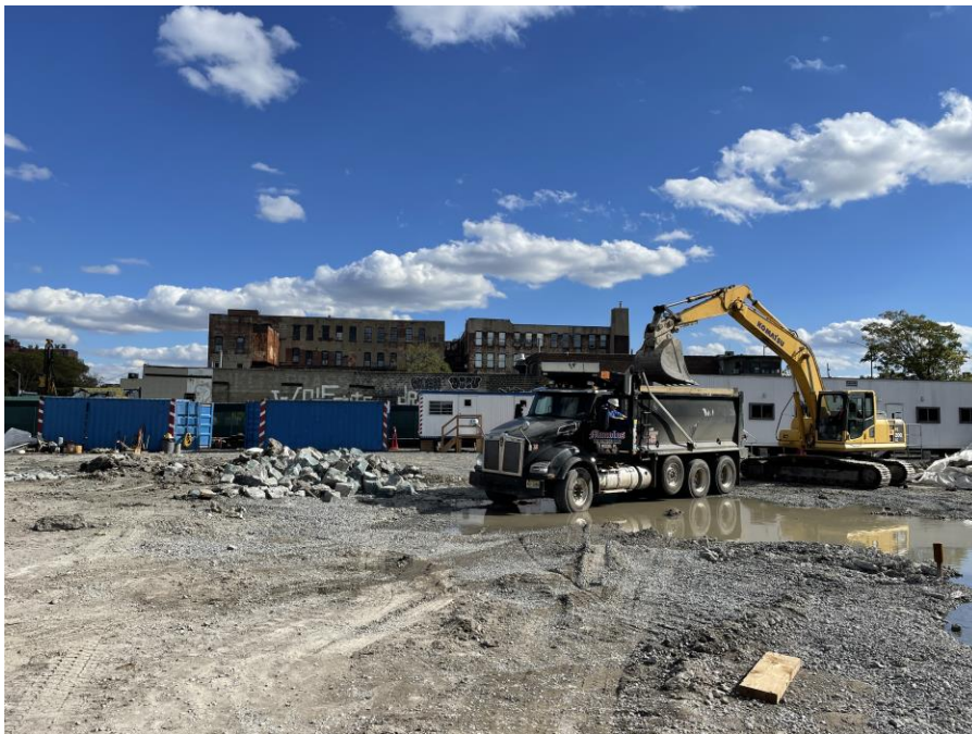
Photo 2: Kingdom loading a permitted tri-axle truck with non-hazardous drilling spoils for off-site disposal from Sackett Place (facing east)
