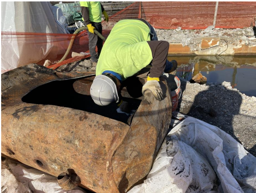
Photo 2: PAL cleaning the UST in the southeastern part of Society Brooklyn (facing west)
