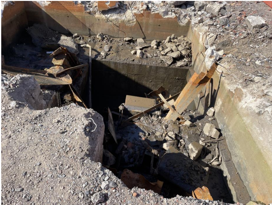
Photo 3: Vault and miscellaneous debris in the southeastern part of Society Brooklyn (facing west)
