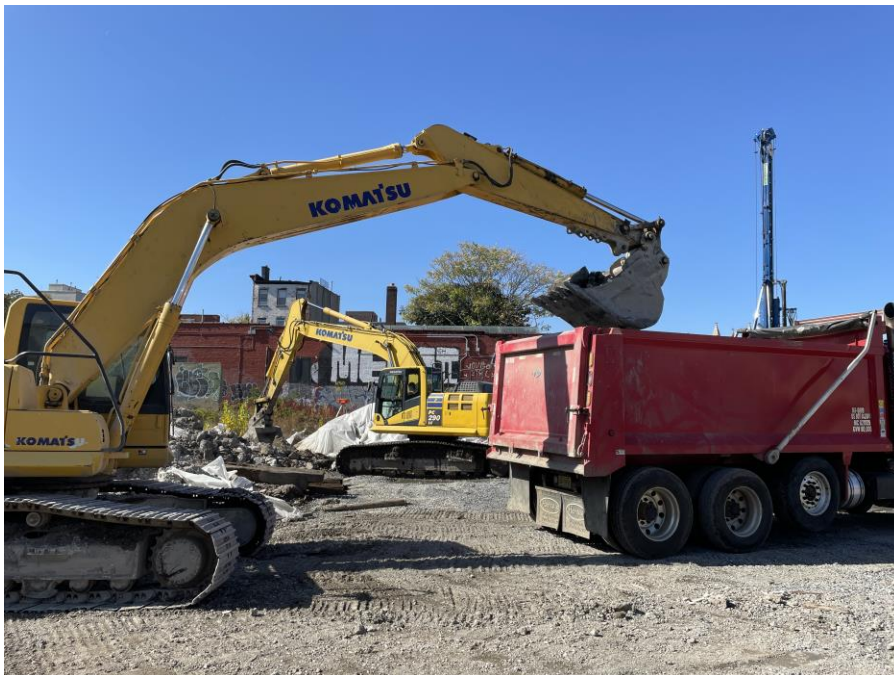
Photo 4: Kingdom loading a permitted tri-axle truck with non-hazardous drilling spoils for off-site disposal from Sackett Place (facing northwest)
