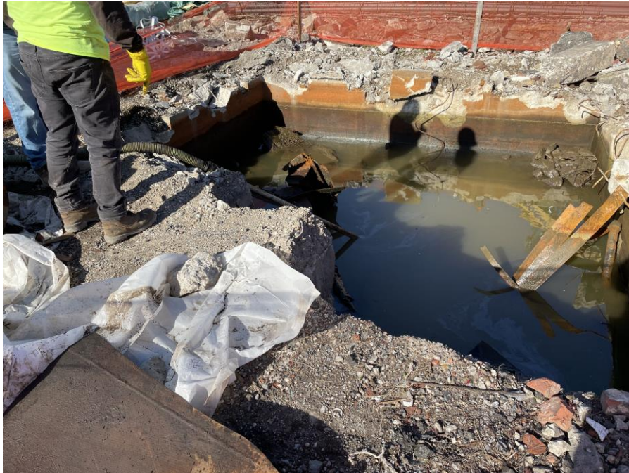
Photo 1: PAL Environmental vacuuming oily water into a permitted truck from the vault in the southeastern part of Society Brooklyn (facing west)
