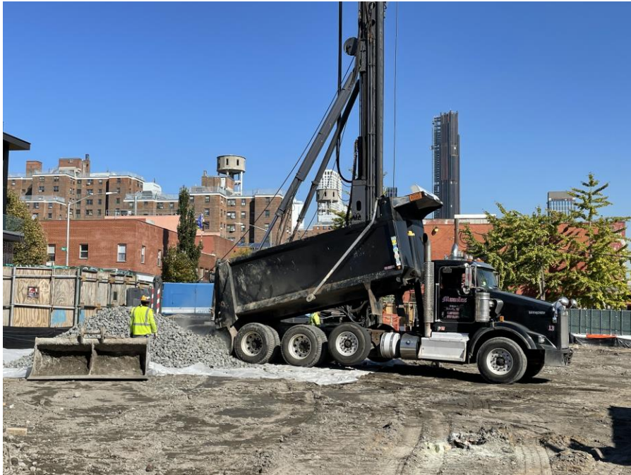
Photo 1: Kingdom importing 2 ½-inch virgin stone from the Stavola Construction Materials Bound Brook quarry in the western part Society Brooklyn (facing north)
