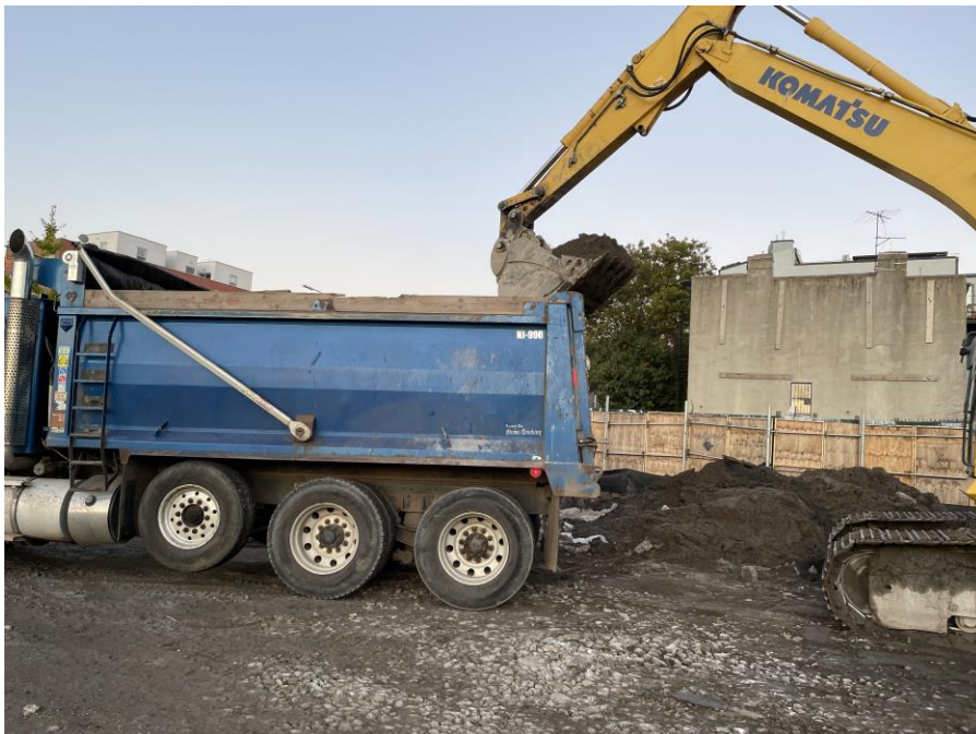
Photo 2: Kingdom loading a permitted tri-axle truck with non-hazardous soil for off-site disposal from Society Brooklyn (facing west)
