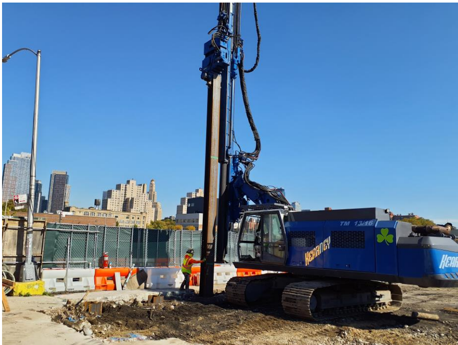
Photo 2: Kingdom installing a soldier pile for the SOE system in the northern part of Sackett Place (facing northeast)
