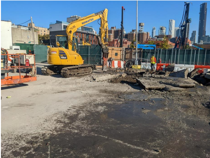
Photo 1: Kingdom demolishing former concrete building slab in the northern part of Sackett Place (facing north)
