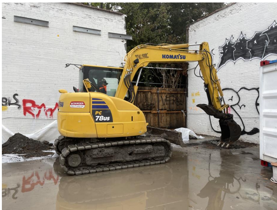
Photo 1: Test pit excavation in the northwestern part of Sackett Place (facing southwest)
