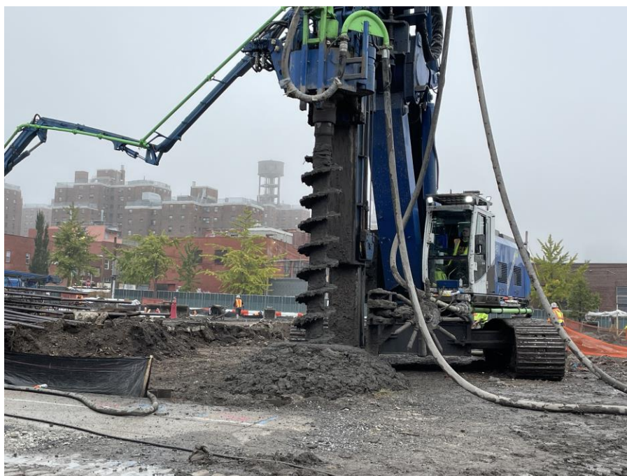
Photo 2: Kingdom installing a foundation pile in the southern part of Society Brooklyn (facing northeast)
