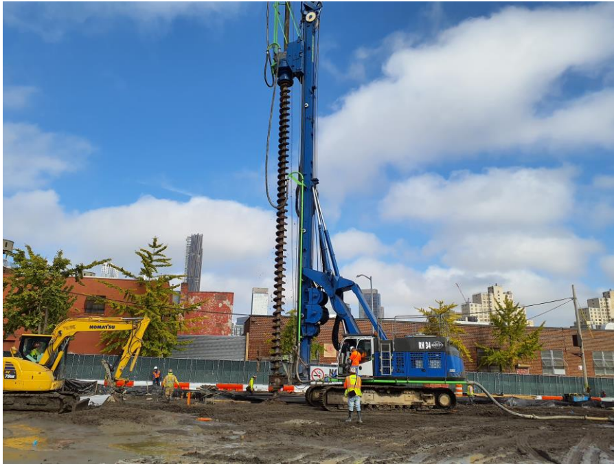
Photo 1: Kingdom installing a foundation pile in the northern part of Society Brooklyn (facing northeast)
