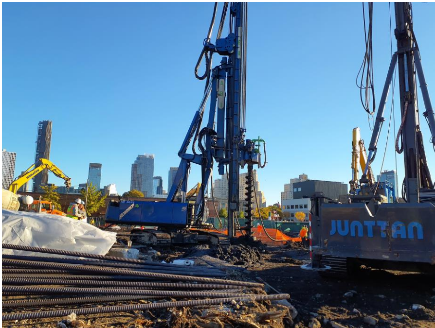
Photo 2: Kingdom installing a foundation pile in the southeastern part of Society Brooklyn (facing north)
