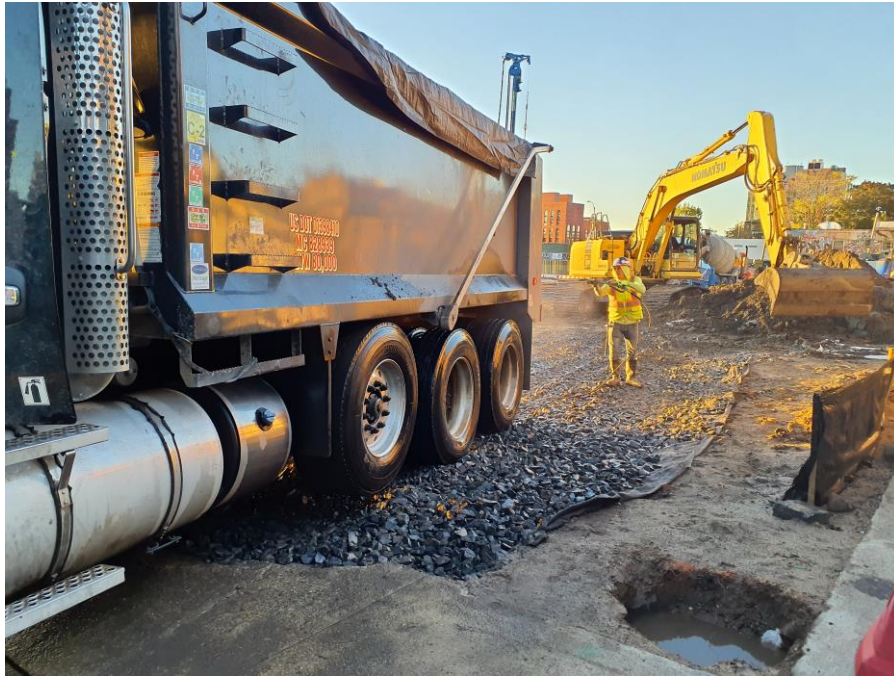
Photo 1: Kingdom washing a permitted tri-axle truck prior to off-site disposal from Society Brooklyn (facing southeast)
