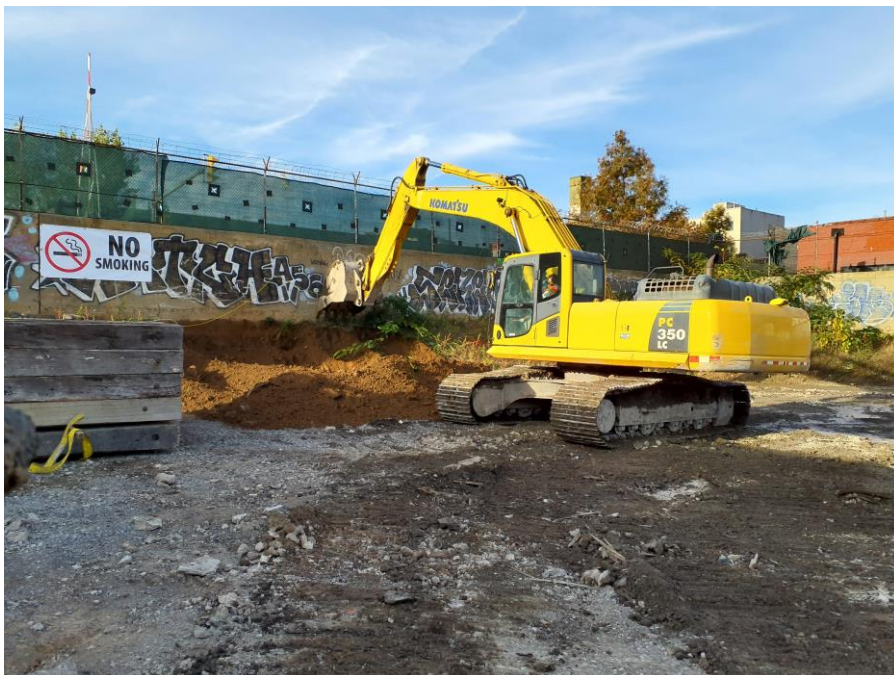
Photo 2: Kingdom excavating bermed historic fill in the southern part of Sackett Place (facing southwest)
