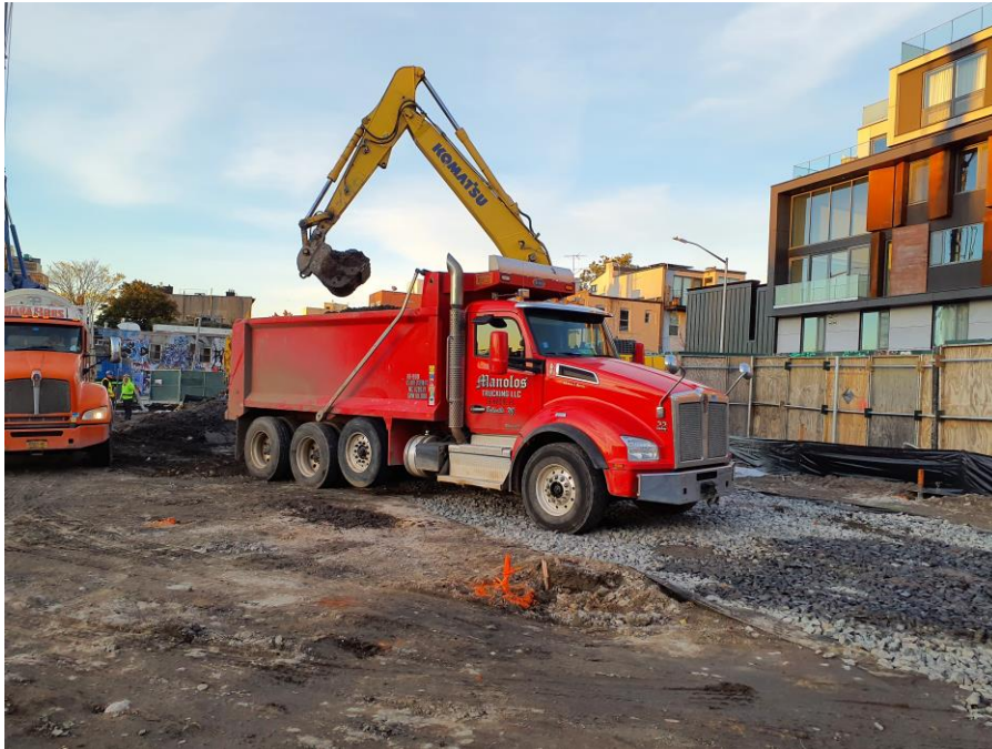
Photo 1: Kingdom loading a permitted tri-axle truck with non-hazardous drilling spoils for off-site disposal from Society Brooklyn (facing southwest)
