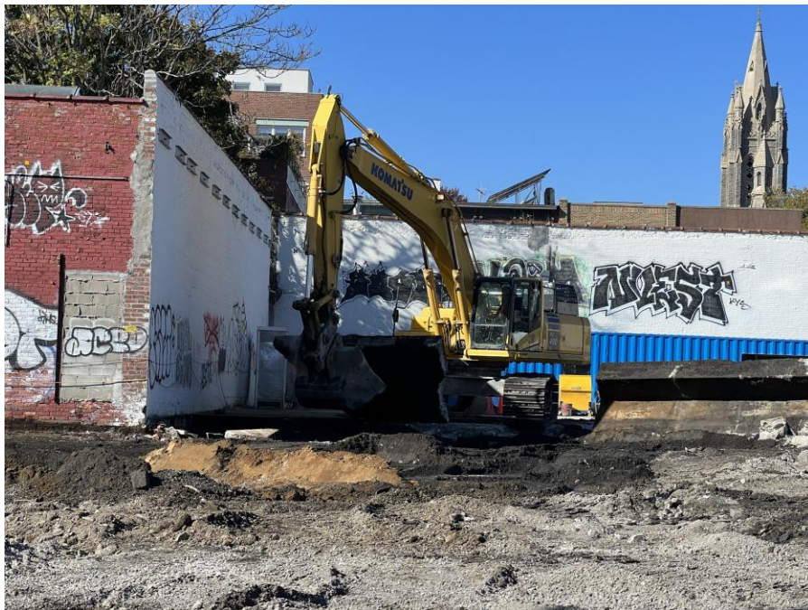
Photo 2: Kingdom demolishing a former concrete building slab in the western part of Sackett Place (facing west)
