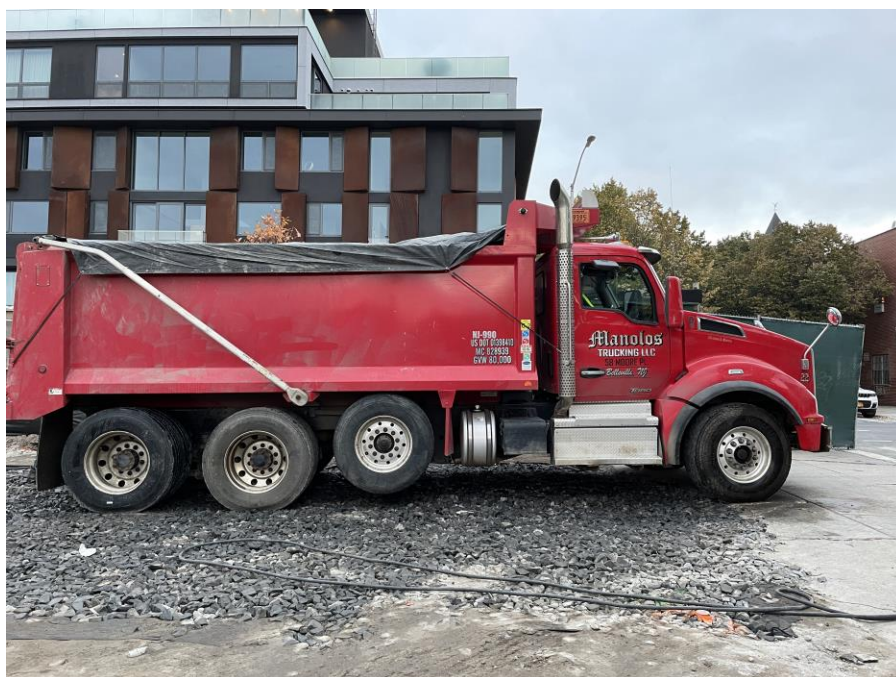
Photo 2: Kingdom exporting non-hazardous soil in a permitted tri-axle truck for off-site disposal from Society Brooklyn (facing northwest)
