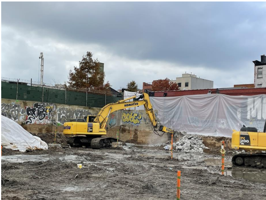
Photo 2: Kingdom demolishing the former concrete building wall in the southwestern part of Sackett Place (facing southwest)
