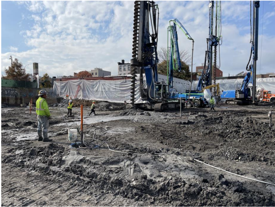
Photo 1: Kingdom installing a foundation pile in the southern part of Sackett Place (facing southwest)
