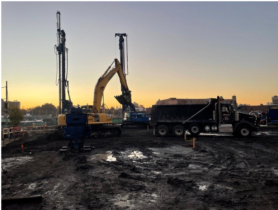
Photo 2: Kingdom exporting non-hazardous soil in a permitted tri-axle truck for off-site disposal from Society Brooklyn (facing east)
