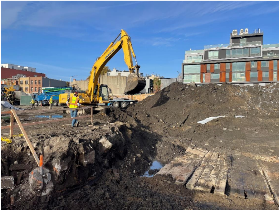
Photo 1: Kingdom installing timber mats in the northern part of Society Brooklyn (facing west)
