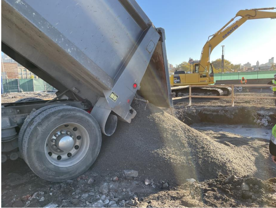
Photo 1: Kingdom imported ½-inch crushed stone from the Impact Environmental Facility in the southeastern part of Society Brooklyn (facing northeast)
