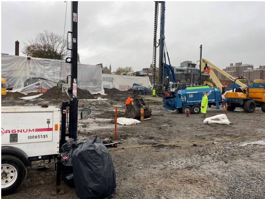
Photo 2: Kingdom installing foundation piles in the northern part of Sackett Place (facing northwest)
