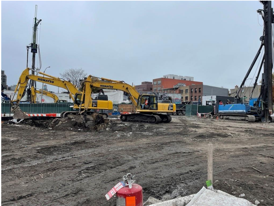
Photo 1: Kingdom excavating in the southern part of Society Brooklyn to install lagging (facing southwest)
