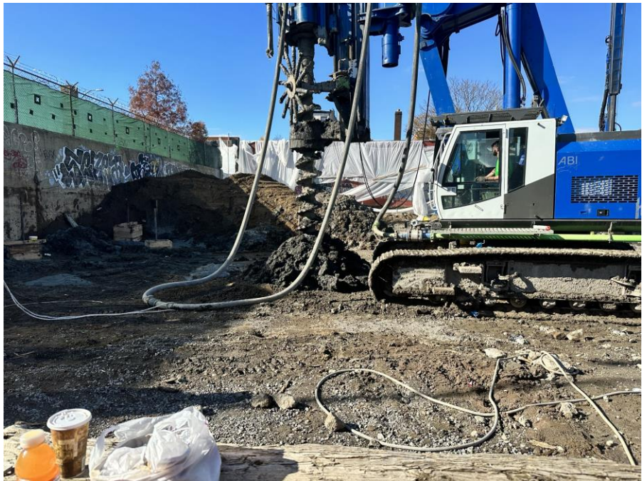
Photo 1: Kingdom installing a foundation pile in the southern part of Sackett Place (facing west)
