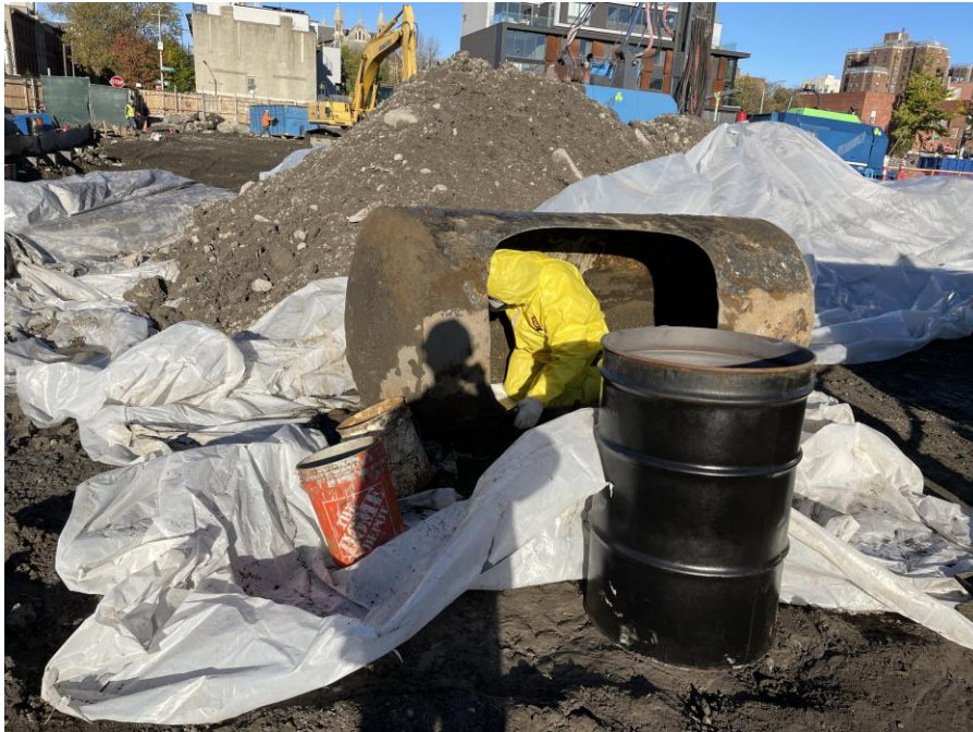
Photo 1: PAL cleaning the UST in the southeastern part of Society Brooklyn (facing northwest)
