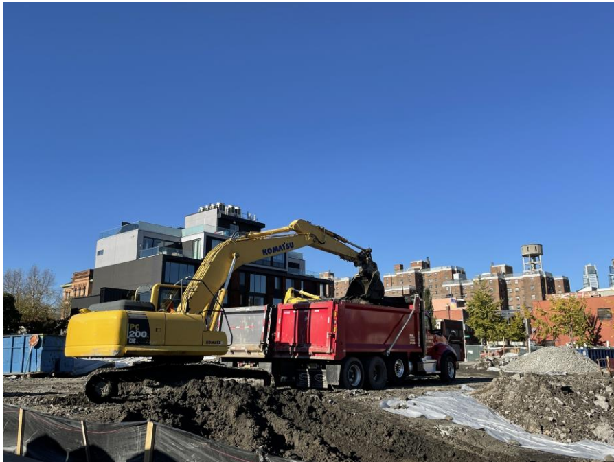
Photo 2: Kingdom loading a permitted tri-axle truck with non-hazardous drilling spoils for off-site disposal from Sackett Place (facing north)
