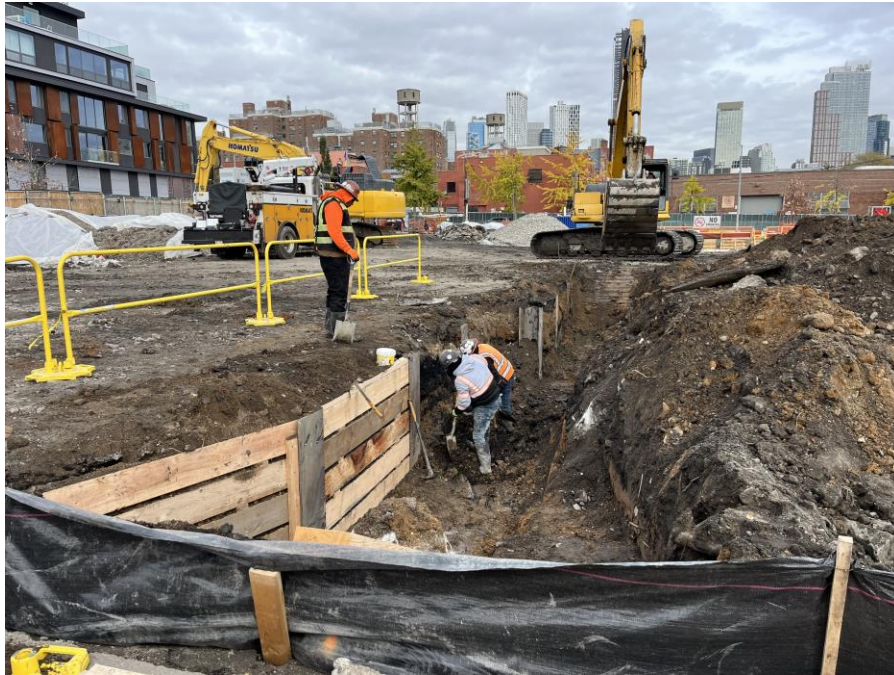
Photo 1: Kingdom installing lagging in the southwestern part of Society Brooklyn (facing north)
