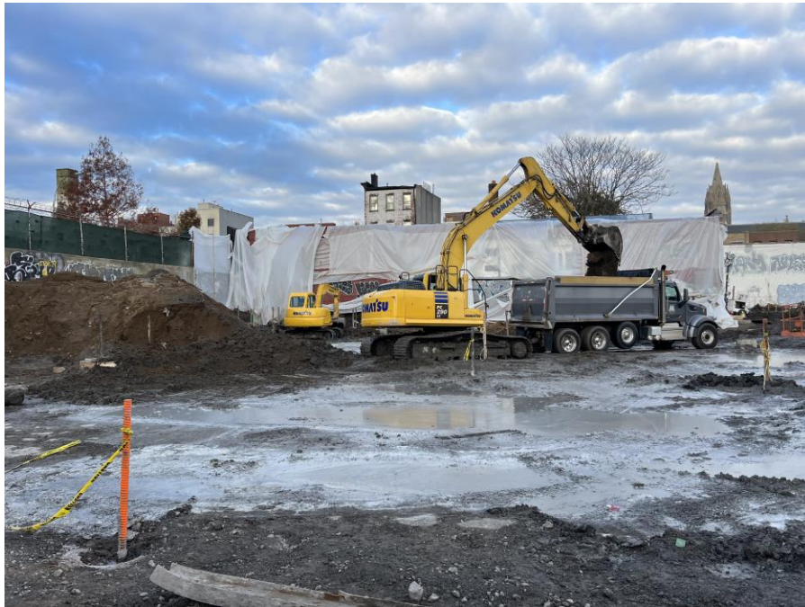
Photo 2: Kingdom loading a permitted tri-axle truck with non-hazardous drilling spoils for off-site disposal from Sackett Place (facing west)
