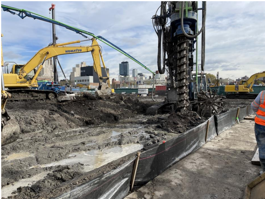
Photo 1: Kingdom installing foundation piles in the southern part of Society Brooklyn (facing east)
