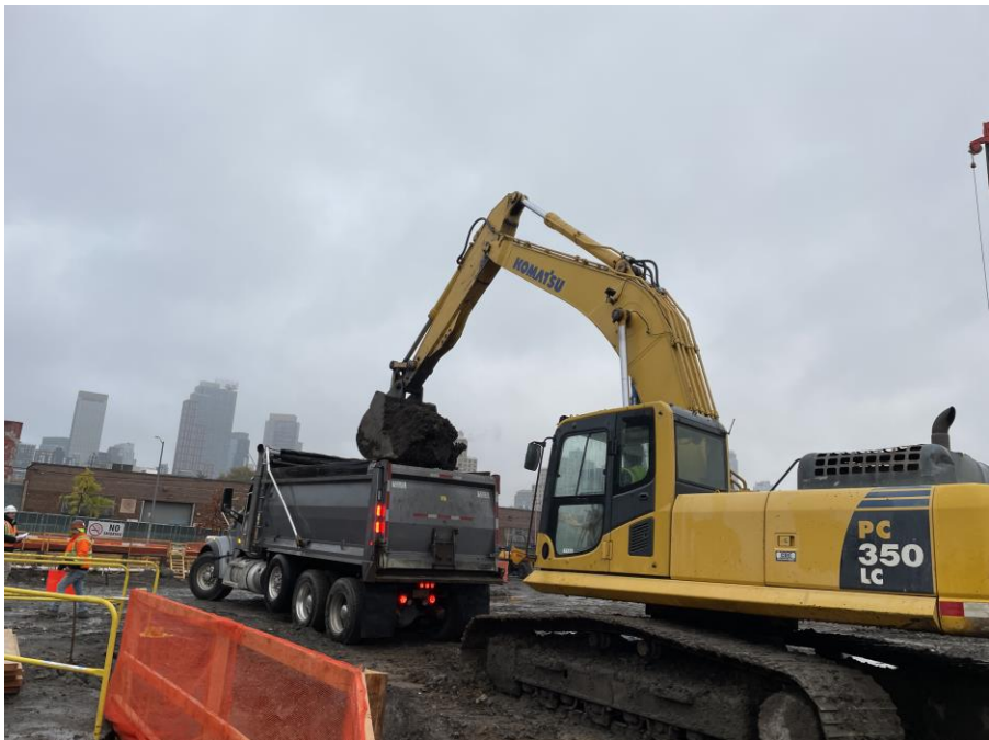
Photo 2: Kingdom loading a permitted tri-axle truck with non-hazardous historic fill for off-site disposal from Society Brooklyn (facing northeast)
