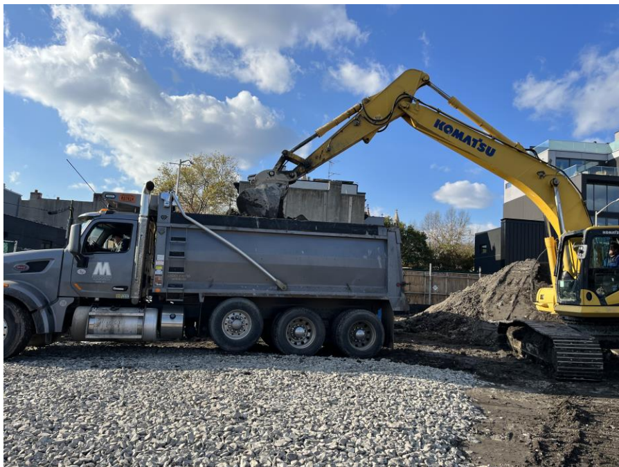
Photo 2: Kingdom loading a permitted tri-axle truck with non-hazardous MGP-impacted drilling spoils for off-site disposal from Society Brooklyn (facing west)
