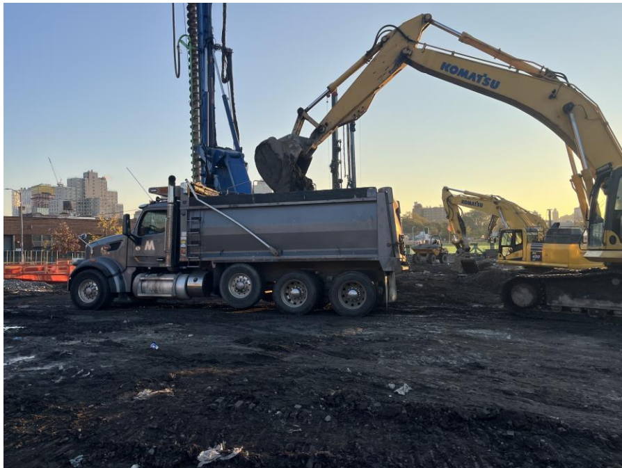
Photo 2: Kingdom loading a permitted tri-axle truck with non-hazardous MGP-impacted drilling spoils for off-site disposal from Society Brooklyn (facing northwest)
