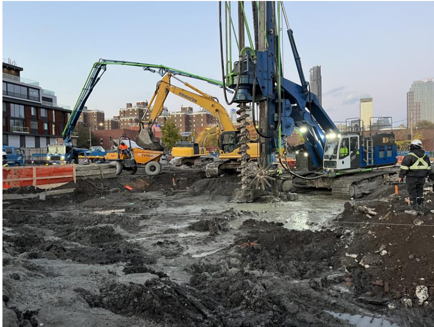
Photo 1: Kingdom installing foundation piles in the southern part of Society Brooklyn (facing northeast)
