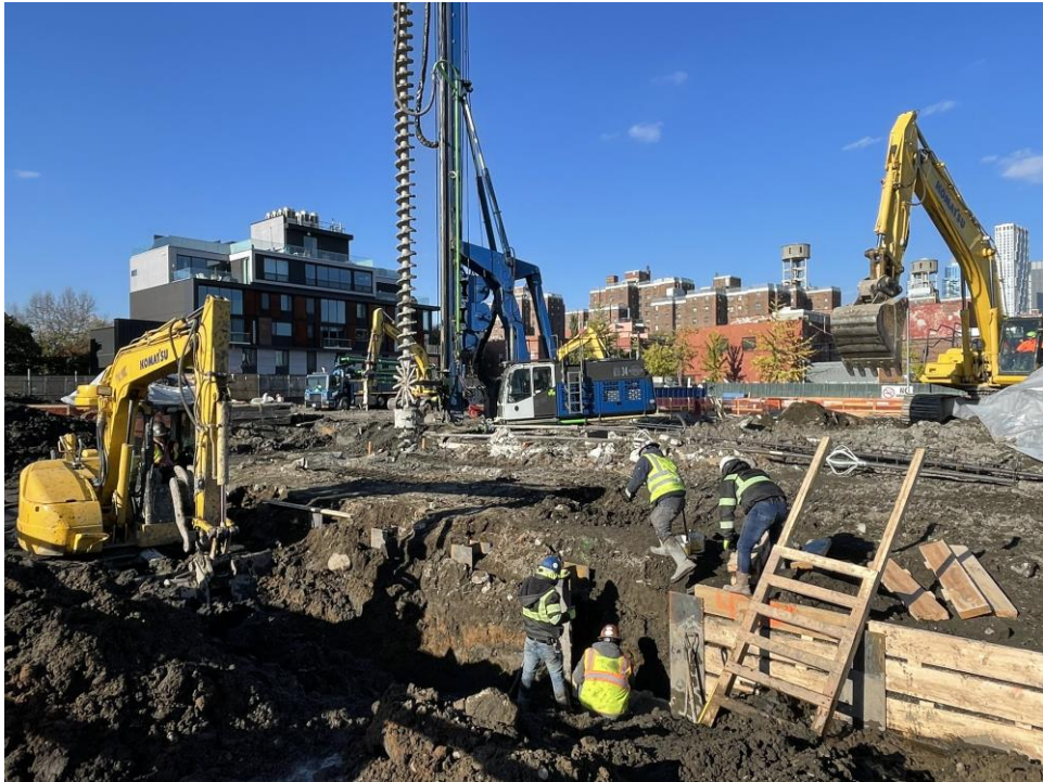
Photo 1: Kingdom installing lagging in the southern part of Society Brooklyn (facing north)
