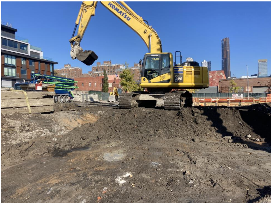
Photo 2: Kingdom excavating hydraulic fluid-impacted soil in the southern part of Society Brooklyn (facing north)
