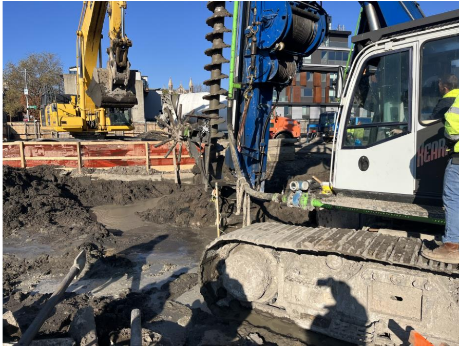
Photo 1: Kingdom installing foundation piles in the southern part of Society Brooklyn (facing west)
