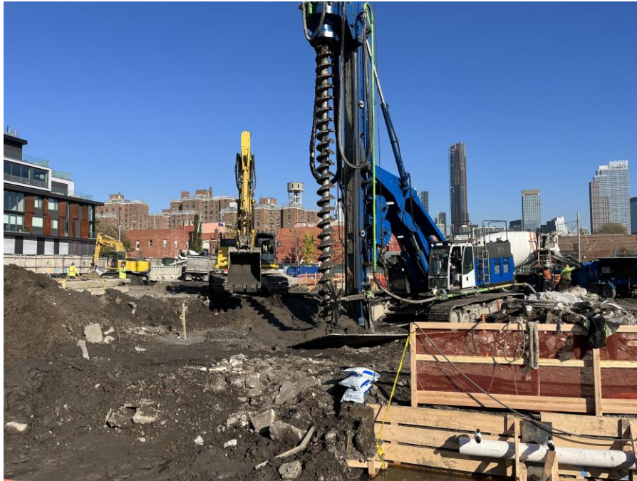
Photo 1: Kingdom installing foundation piles in the southern part of Society Brooklyn (facing north)
