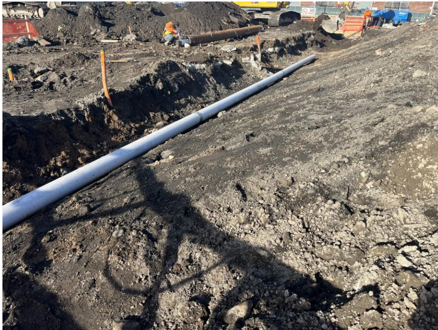
Photo 2: Kingdom installing dewatering piping for the dewatering system in the central part of Society Brooklyn (facing northwest)
