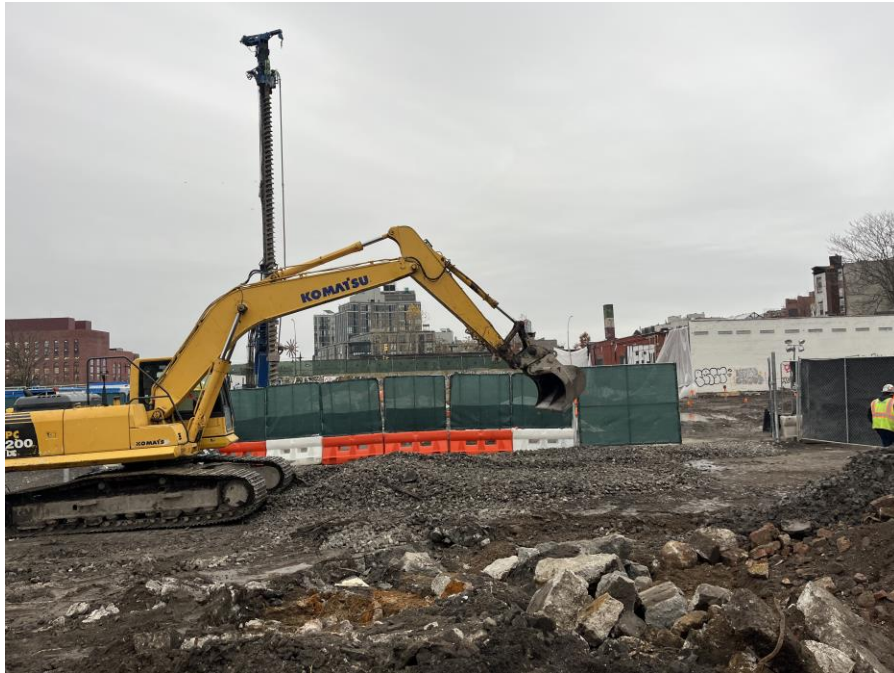
Photo 1: Kingdom repairing the truck tracking pad in the southeastern part of Society Brooklyn (facing south)
