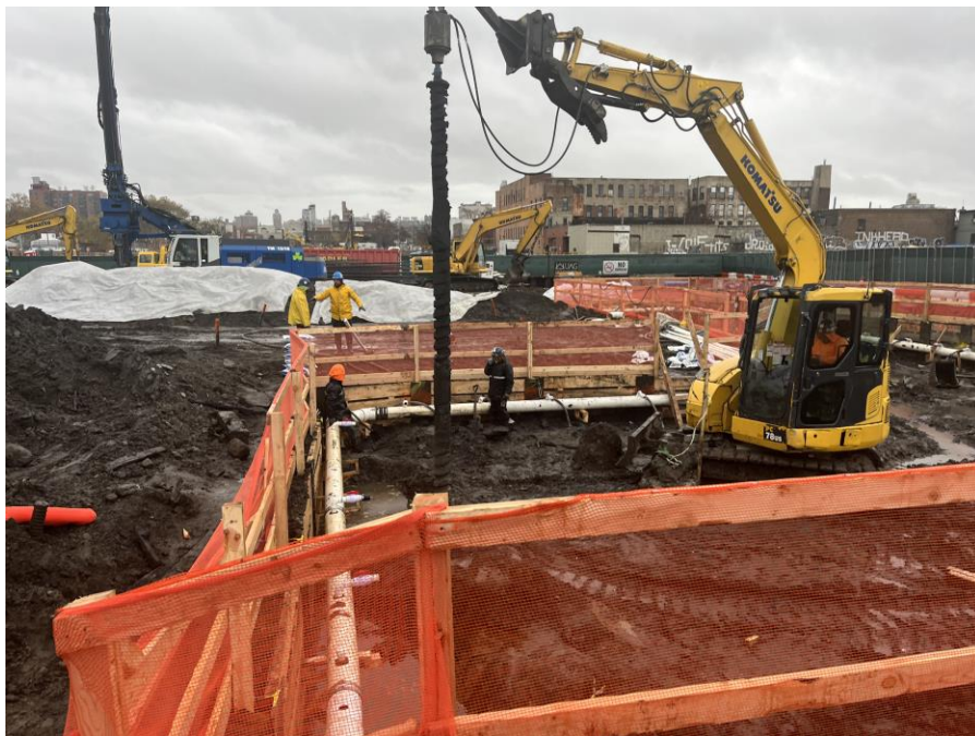
Photo 2: Kingdom installing dewatering wells for the dewatering system in the southern part of Society Brooklyn (facing east)
