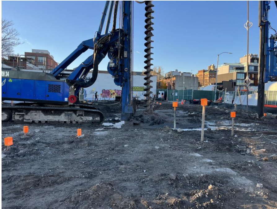
Photo 1: Kingdom installing foundation piles in the northern part of Sackett Place (facing west)
