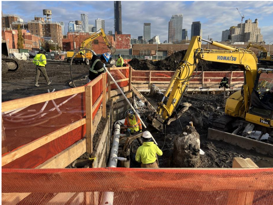
Photo 2: Kingdom installing dewatering wells for the dewatering system in the southern part of Society Brooklyn (facing north)
