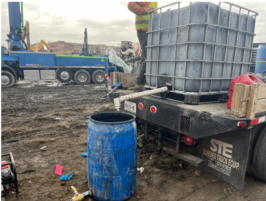
Photo 4: Lakewood Environmental mixing Petrofix injectate in the western part of Society Brooklyn (facing east)
