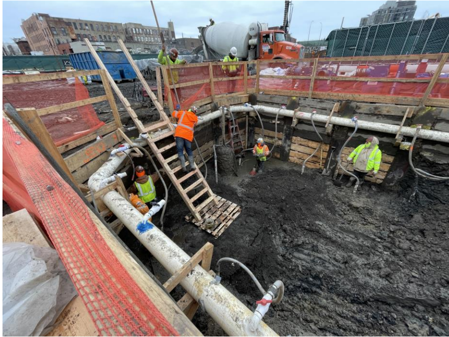
Photo 1: Kingdom installing lagging in the southern part of Society Brooklyn (facing northeast)
