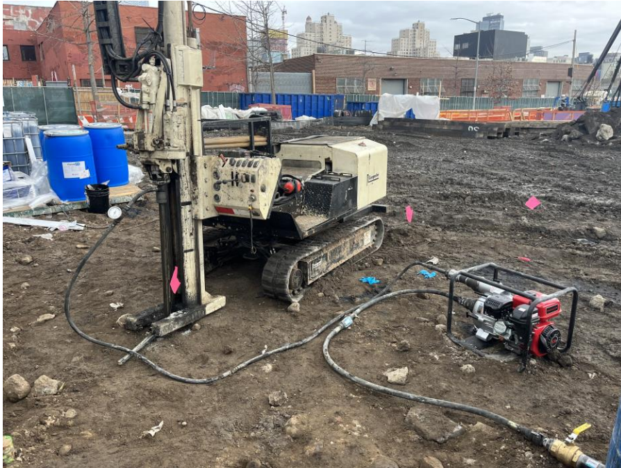
Photo 3: Lakewood Environmental implementing in-situ groundwater remediation via direct-push remedial injections in the western part of Society Brooklyn (facing northeast)
