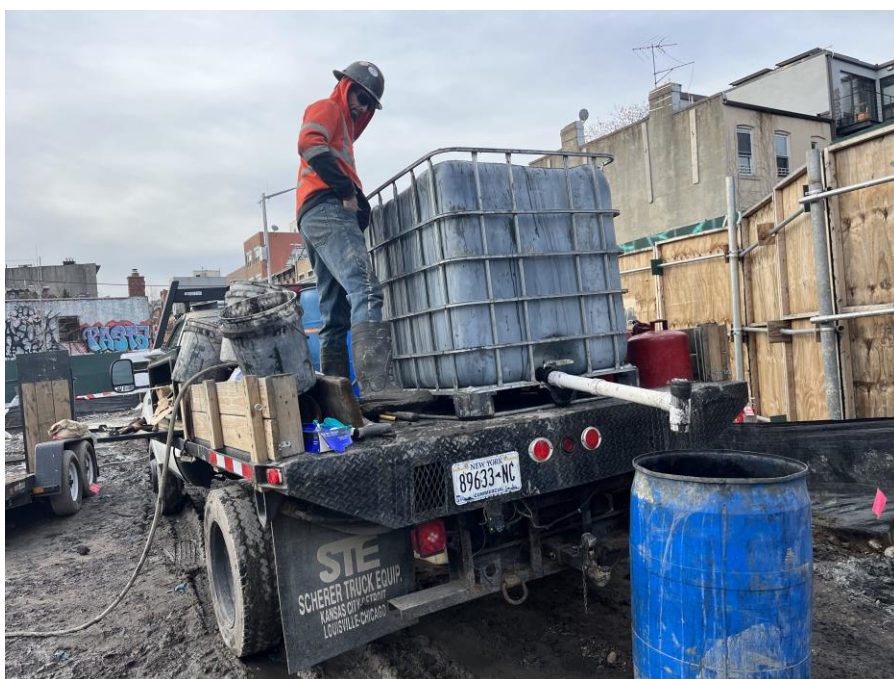
Photo 4: Lakewood Environmental mixing Petrofix for remedial injections in the western part of Society Brooklyn (facing southwest)
