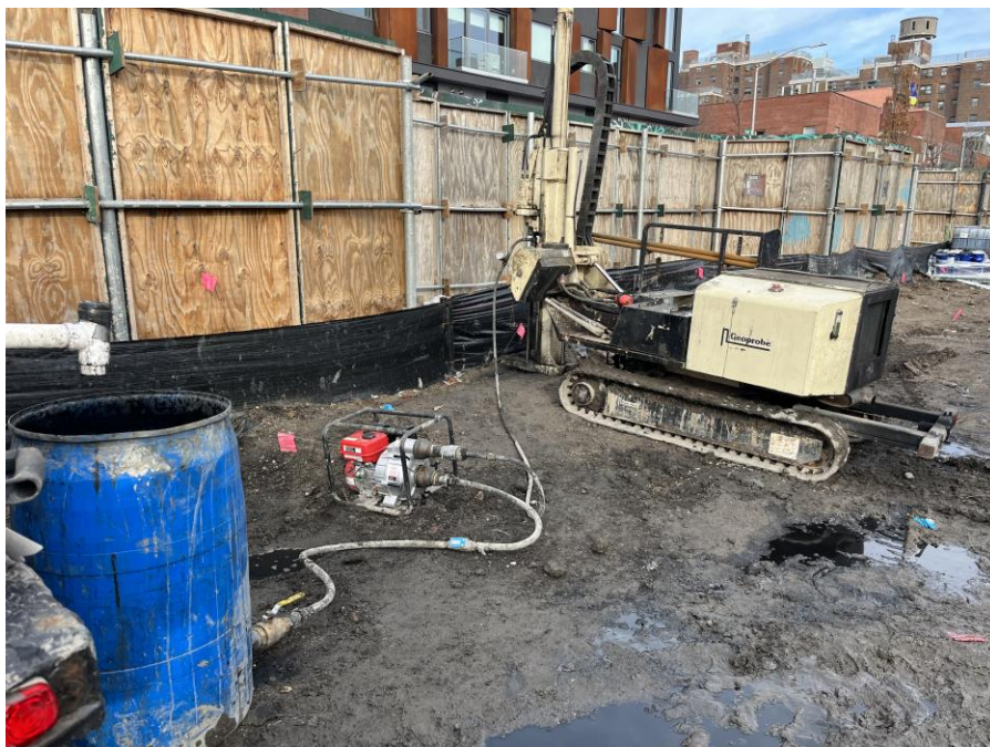
Photo 3: Lakewood Environmental implementing in-situ groundwater remediation via direct-push remedial injections in the western part of Society Brooklyn (facing northwest)
