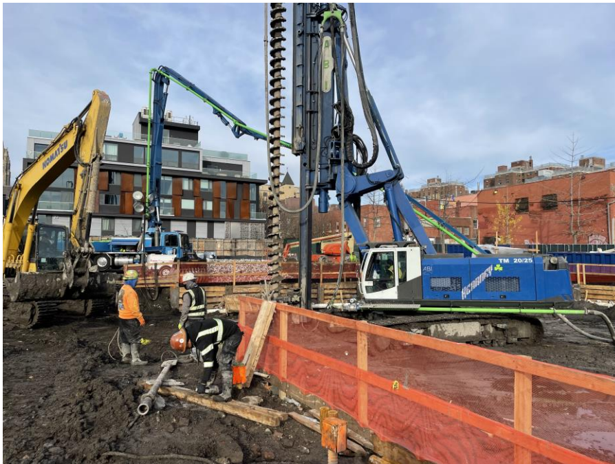
Photo 2: Kingdom installing foundation piles in the northern part of Society Brooklyn (facing north)
