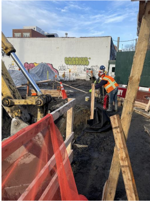
Photo 1: Kingdom applying Biosolve Pinkwater during excavation in the northern part of Society Brooklyn (facing west)
