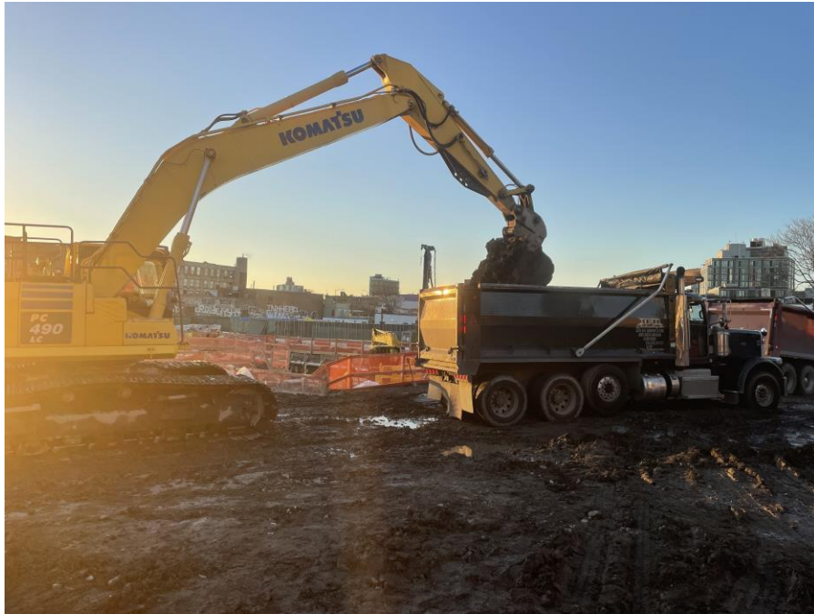
Photo 1: Kingdom loading a permitted tri-axle truck truck with non-hazardous drilling spoils and historic fill for off-site disposal from Society Brooklyn (facing southeast)
