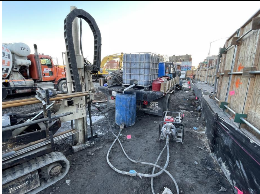
Photo 3: Lakewood Environmental implementing in-situ groundwater remediation via direct-push remedial injections in the western part of Society Brooklyn (facing south)
