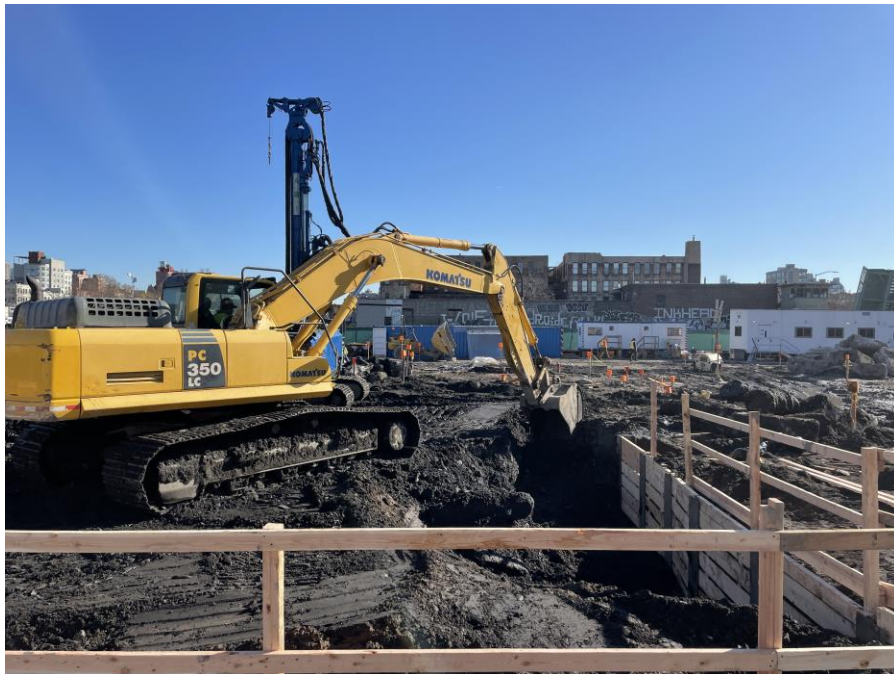
Photo 2: Kingdom excavating in the northern part of Sackett Place to install lagging (facing east)
