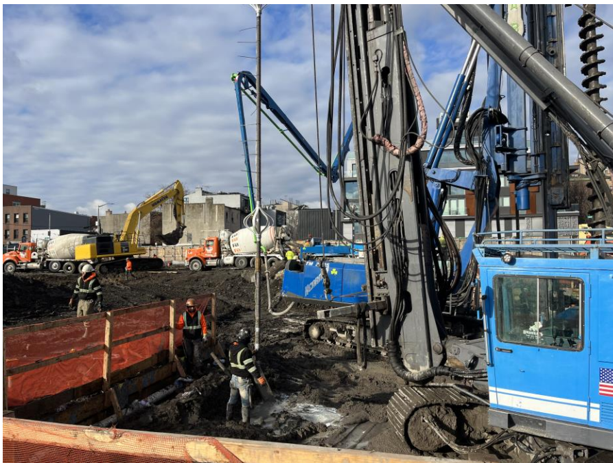
Photo 2: Kingdom installing foundation piles in the northern part of Society Brooklyn (facing southwest)
