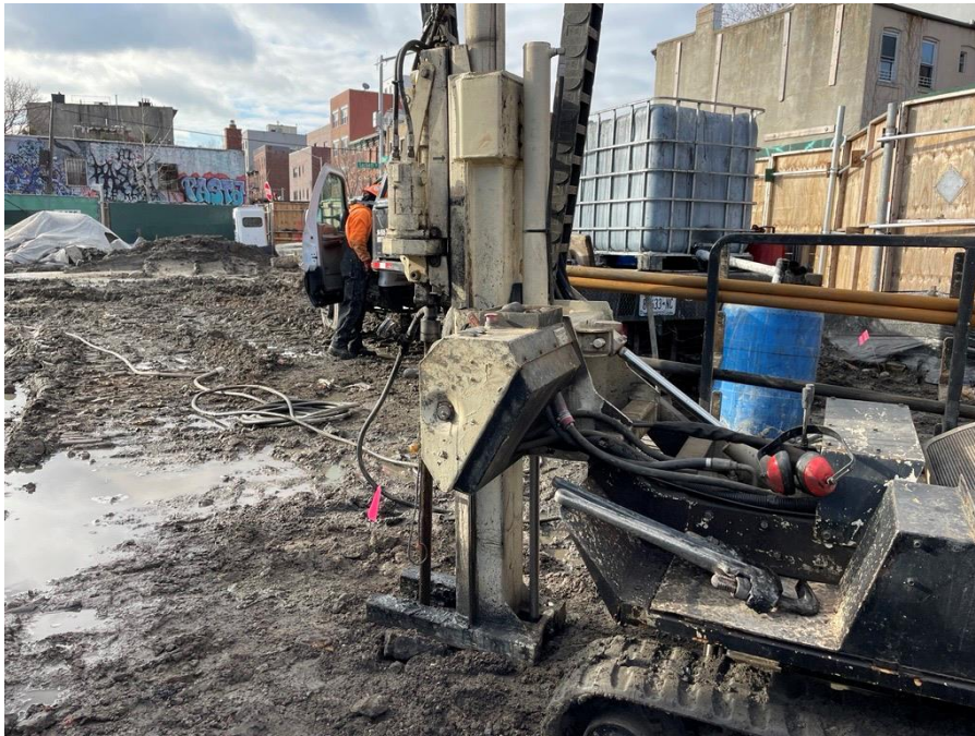
Photo 3: Lakewood Environmental implementing in-situ groundwater remediation via direct-push remedial injections in the western part of Society Brooklyn (facing southwest)
