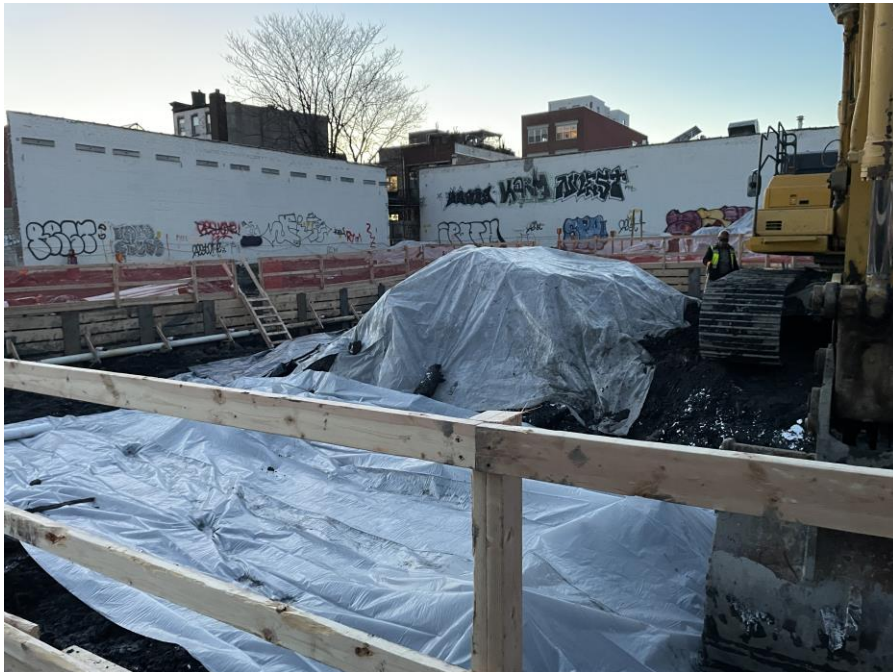
Photo 2: Kingdom covering the base of the excavation in the northern part of Sackett Place with polyethylene sheeting (facing southwest)
