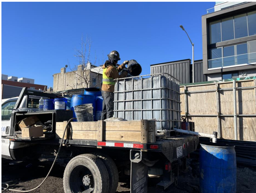
Photo 4: Lakewood Environmental mixing Petrofix for remedial injections in the western part of Society Brooklyn (facing west)
