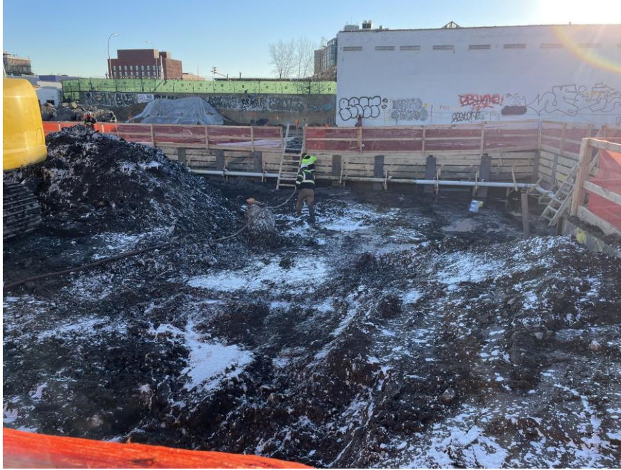
Photo 1: Kingdom applying ATMOS odor suppressant foam in the northern part of Sackett Place (facing south)
