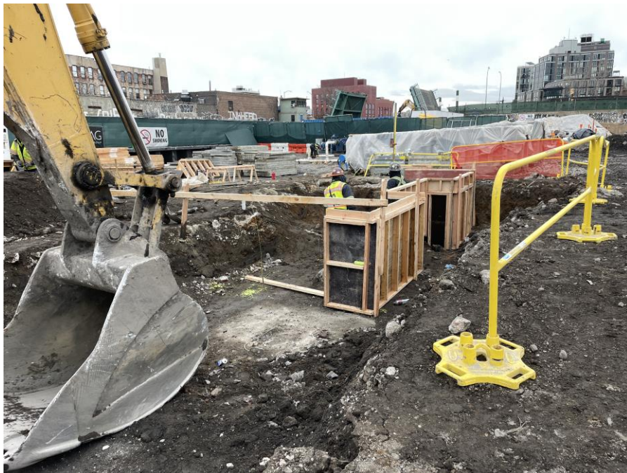
Photo 2: Kingdom installing formwork for pile caps in the eastern part of Society Brooklyn (facing southeast)
