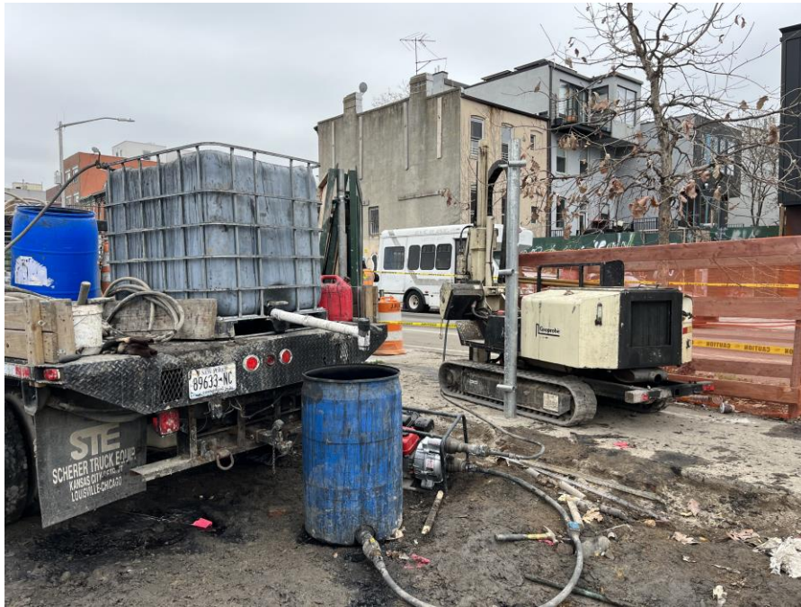
Photo 3: Lakewood Environmental implementing in-situ groundwater remediation via direct-push remedial injections in the west-adjointing Bond Street sidewalk (facing southwest)
