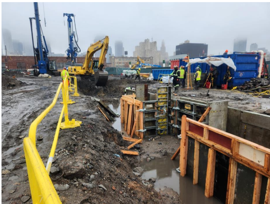
Photo 2: Kingdom excavating to install formwork for pile caps in the eastern part of Society Brooklyn (facing northeast)
