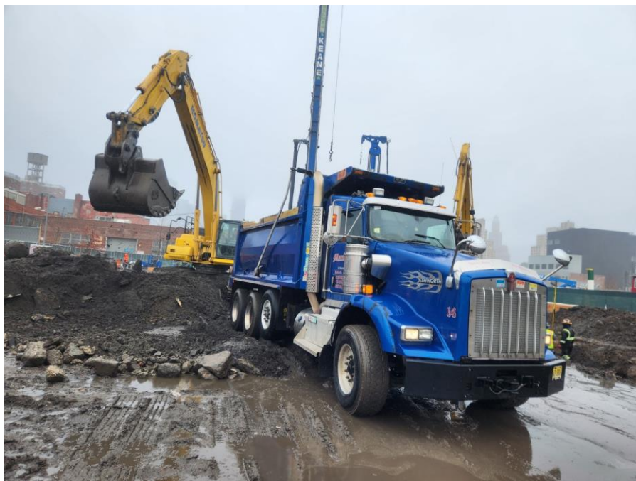
Photo 1: Kingdom loading a permitted tri-axle truck with non-hazardous drilling spoils and historic fill for off-site disposal from Society Brooklyn (facing northeast)
