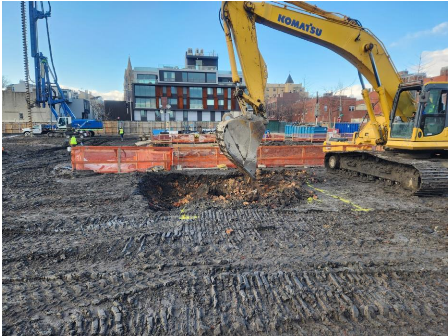
Photo 2: Kingdom excavating to install formwork for pile caps in the northern part of Society Brooklyn (facing northwest)
