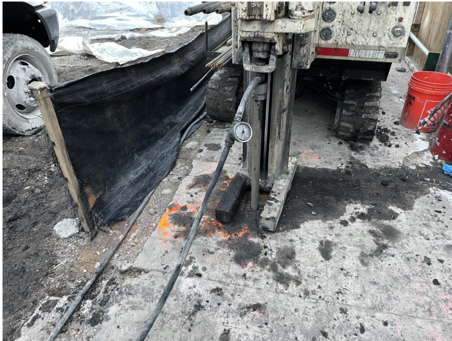
Photo 3: Lakewood Environmental implementing in-situ groundwater remediation via direct-push remedial injections in the west-adjointing Bond Street sidewalk (facing south)
