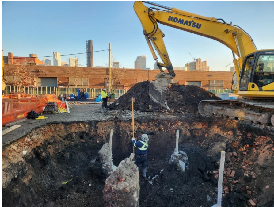
Photo 1: Kingdom excavating to install formwork for pile caps in the northeastern part of Society Brooklyn (facing northeast)
