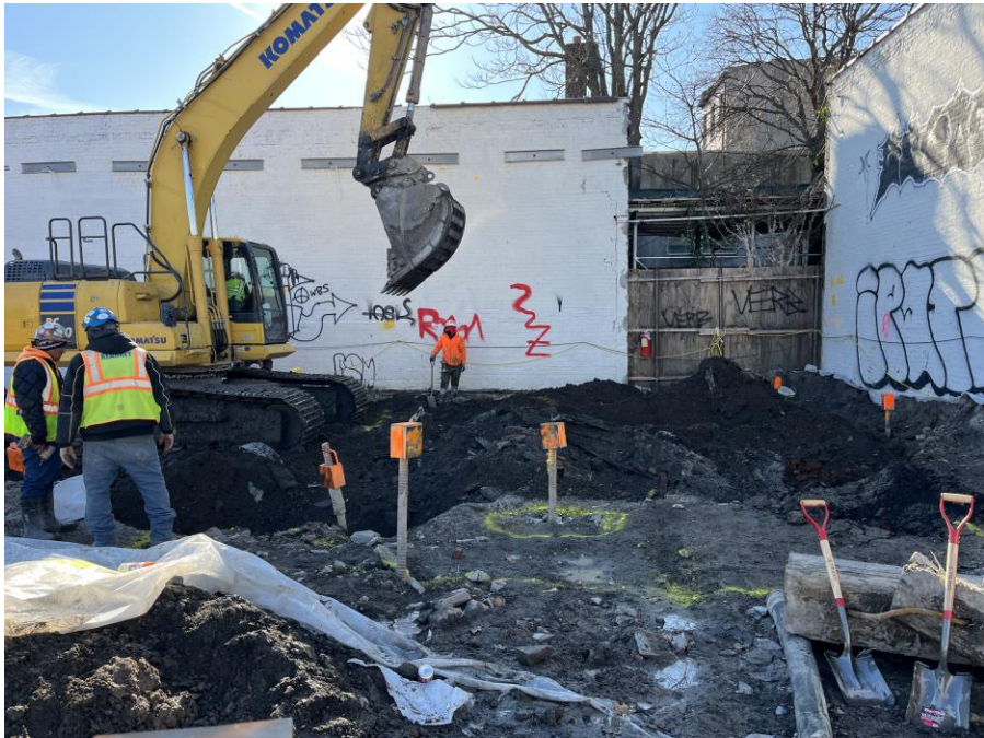
Photo 1: Kingdom excavating to install formwork for pile caps in the western part of Sackett Place (facing south)
