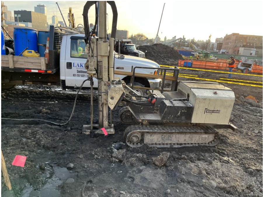
Photo 3: Lakewood Environmental implementing in-situ groundwater remediation via direct-push remedial injections in the western part of Society Brooklyn (facing east)
