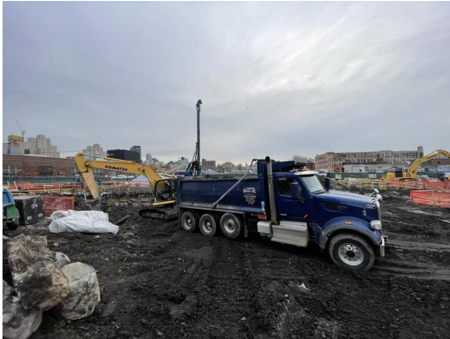
Photo 1: Kingdom live-loading a permitted tri-axle truck with non-hazardous soil and historic fill for off-site disposal from Society Brooklyn (facing northeast)
