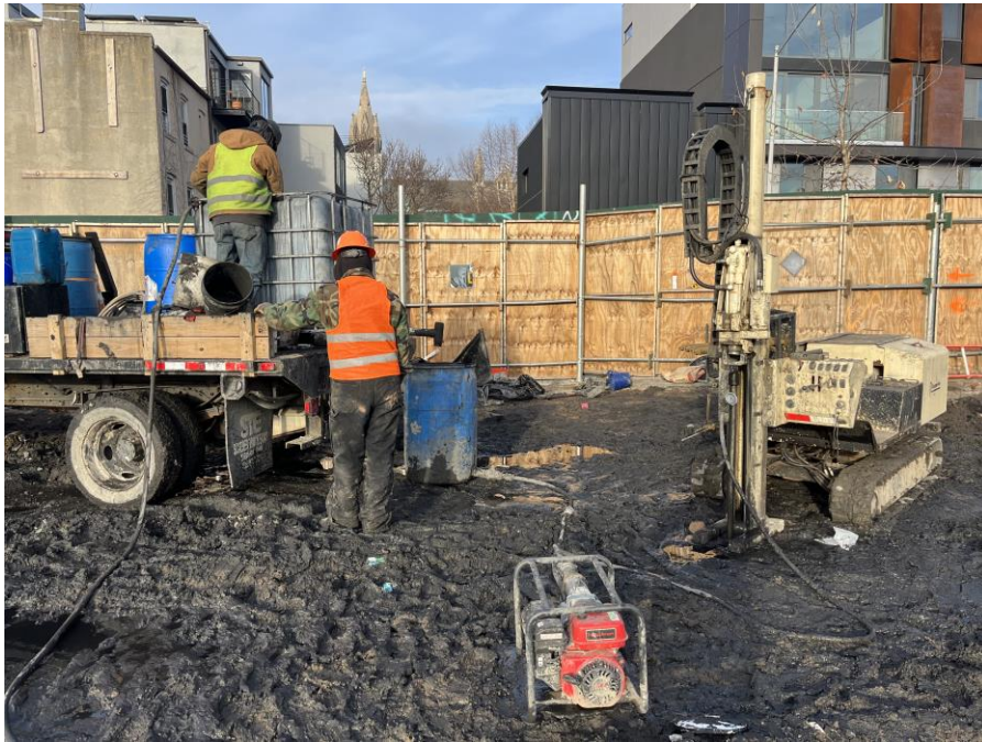
Photo 3: Lakewood Environmental implementing in-situ groundwater remediation via direct-push remedial injections in the western part of Society Brooklyn (facing west)
