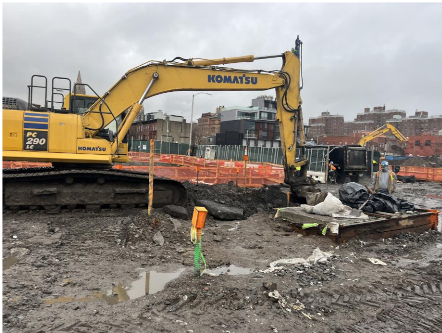
Photo 2: Kingdom excavating in the northeastern part of Sackett Place for pile cap load testing (facing north)
