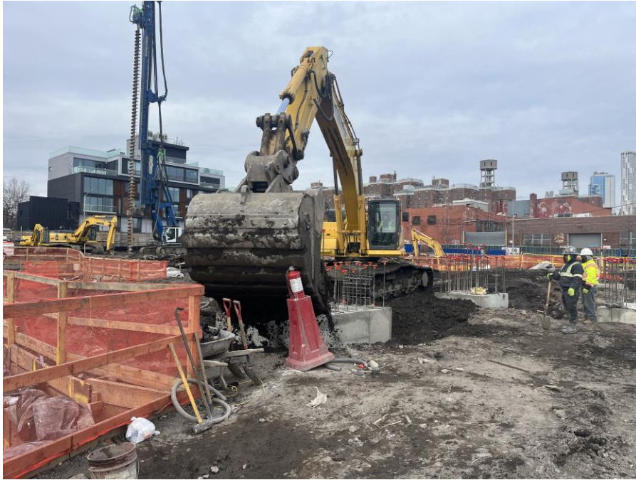
Photo 1: Kingdom backfilling around pile caps in the eastern part of Society Brooklyn (facing north)
