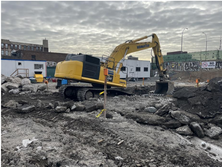
Photo 2: Kingdom excavating for pile cap load testing in the southern part of Sackett Place (facing southeast)
