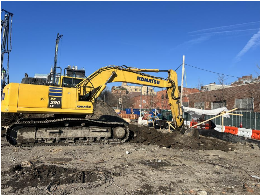
Photo 2: Kingdom excavating for structural pile cap load testing in the northeastern part of Society Brooklyn (facing northwest)
