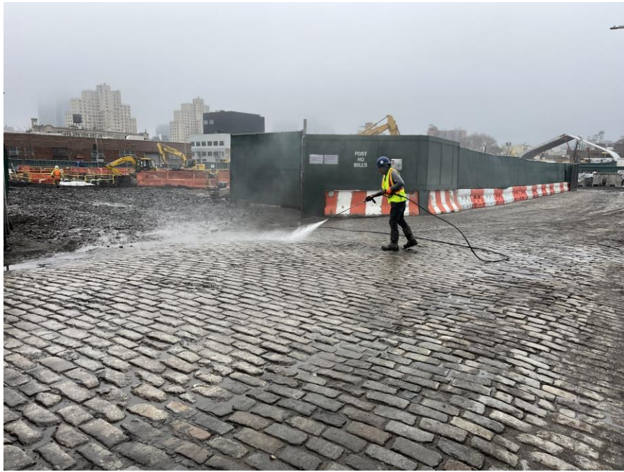
Photo 3: Kingdom cleaning sediment out of Sackett Street (facing northeast)
