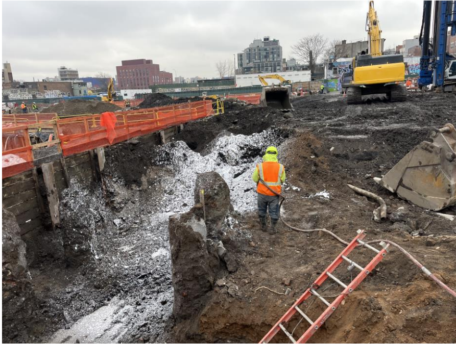
Photo 1: Kingdom applying ATMOS odor suppressing foam in the western part of Remedial Excavation Area No. 1 in the northern part of Society Brooklyn (facing southeast)
