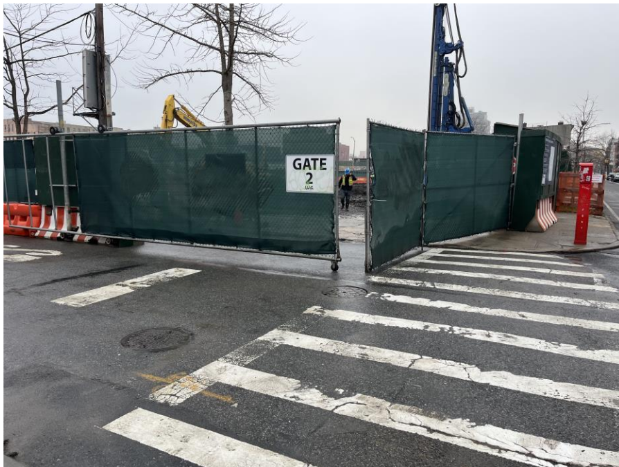
Photo 4: View of site entrance in the northwestern part of Society Brooklyn (facing south)
