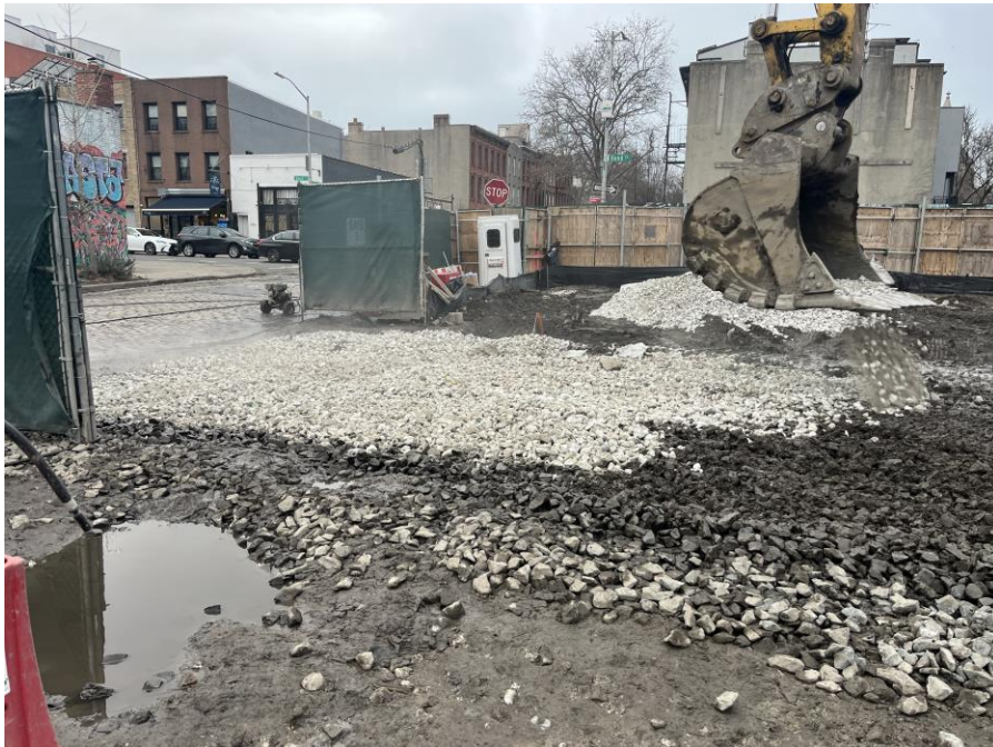
Photo 2: Kingdom repairing the stabilized construction entrance with 2.5-inch stone in the southwestern part of Society Brooklyn (facing southwest)
