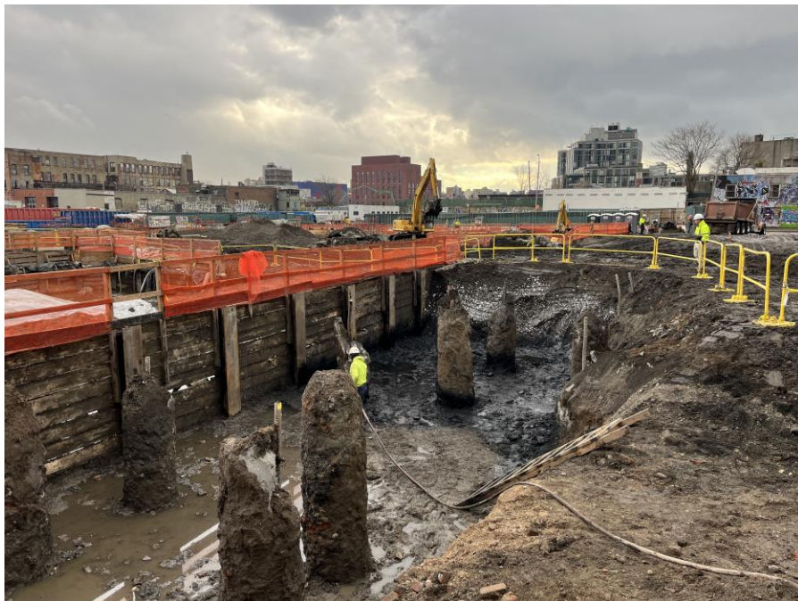
Photo 2: Kingdom applying Petrofix reagent to the base and sidewalls of the western part of Remedial Excavation Area No. 1 in the northern part of Society Brooklyn (facing south)
