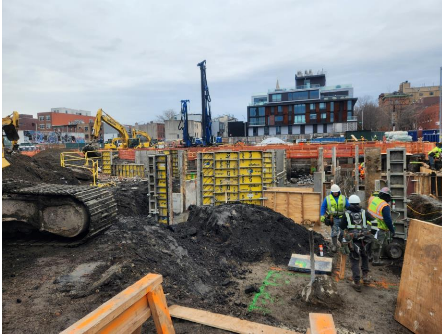
Photo 1: Kingdom installing pile cap formwork in the northeastern part of Society Brooklyn (facing west)
