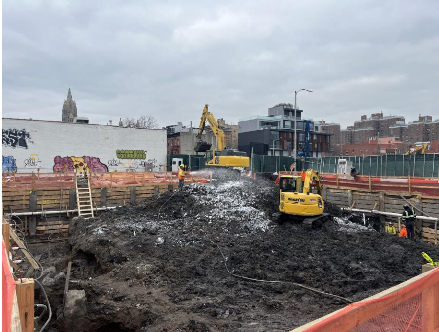
Photo 1: Kingdom applying ATMOS odor suppressing foam in the northern part of Sackett Place (facing northwest)
