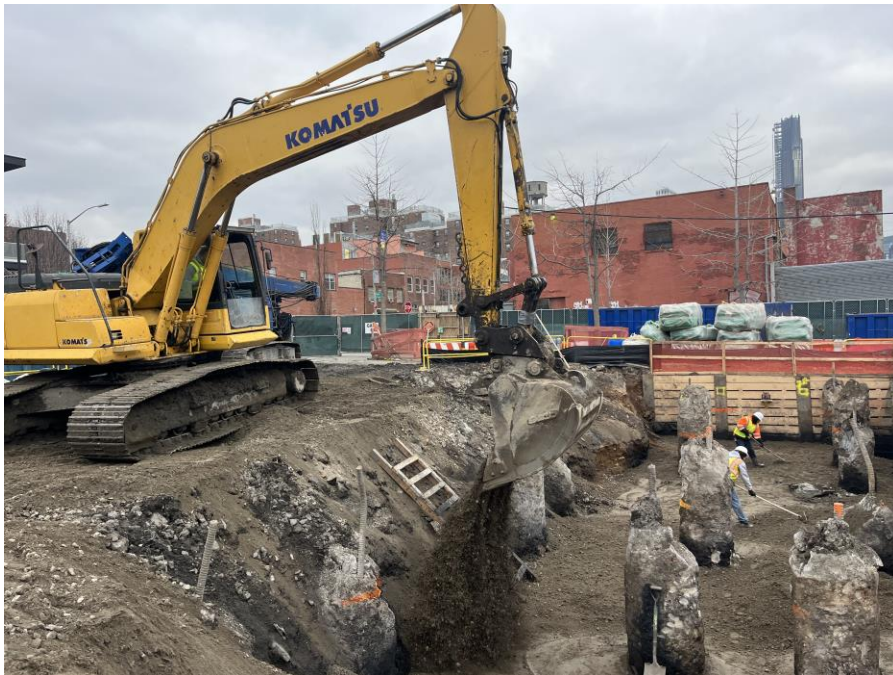
Photo 2: Kingdom backfilling with 0.5-inch crushed stone in the northern part of Society Brooklyn (facing north)
