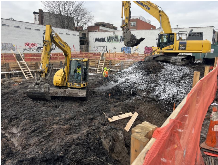
Photo 1: Kingdom applying ATMOS odor suppressing foam in the northern part of Sackett Place (facing southwest)
