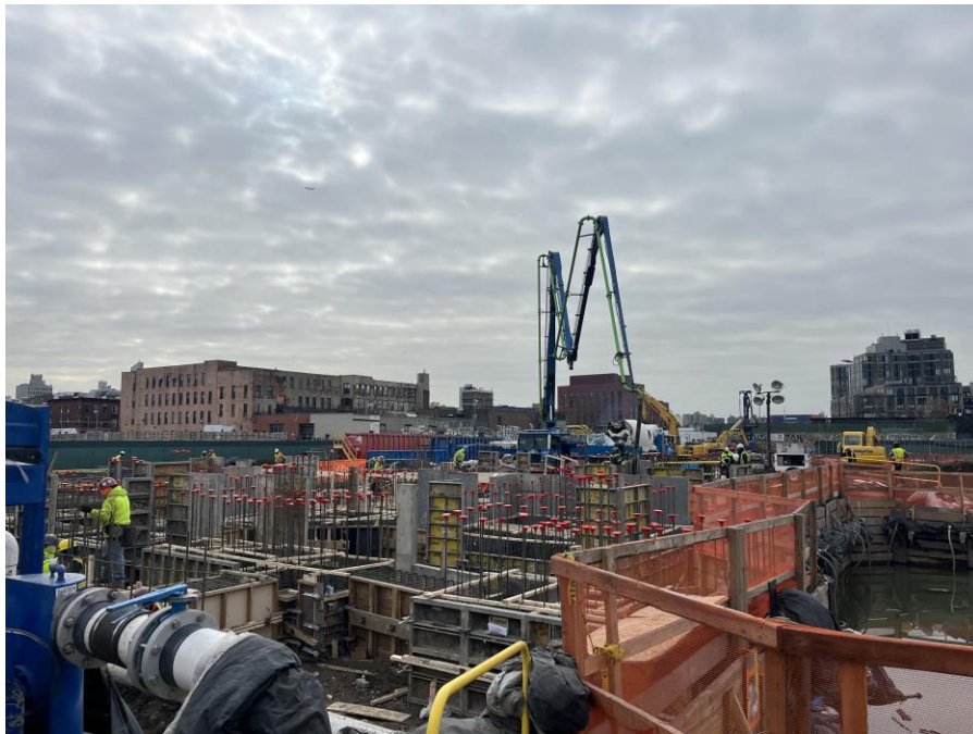
Photo 2: Kingdom pouring concrete for foundation elements in the northern part of Society Brooklyn (facing southeast)
